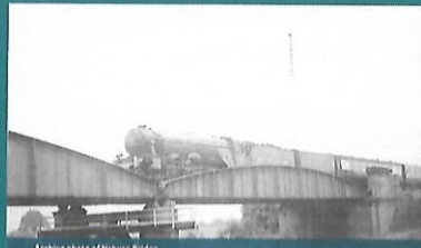
Archive photo of Naburn Bridge.
