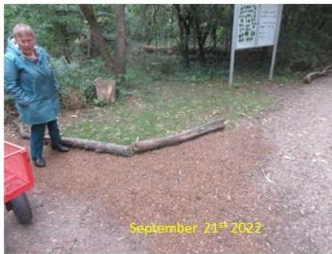
Levelling path with pea gravel after weeding, leaf removal and restoring path edges.
